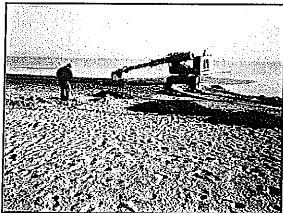
Muck removal at BCSRA in 1992
