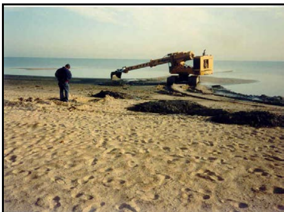
Muck removal at BCSRA in 1992
