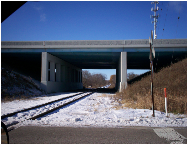
Looking west at the Rail line at I-75
